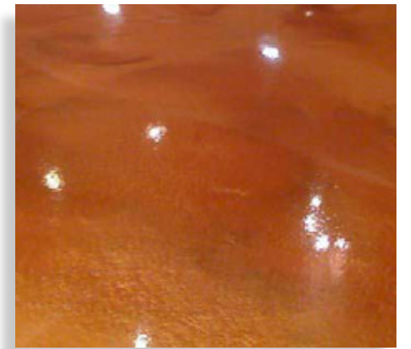
STAINED CONCRETE FLOORS
